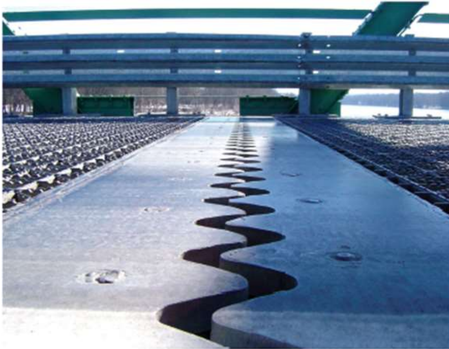
Figure 6: Expansion joint on a bridge
