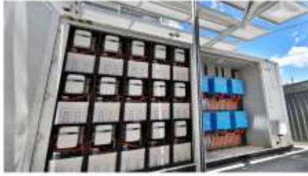
Commercial flow batteries, such as this zinc-bromine system.
